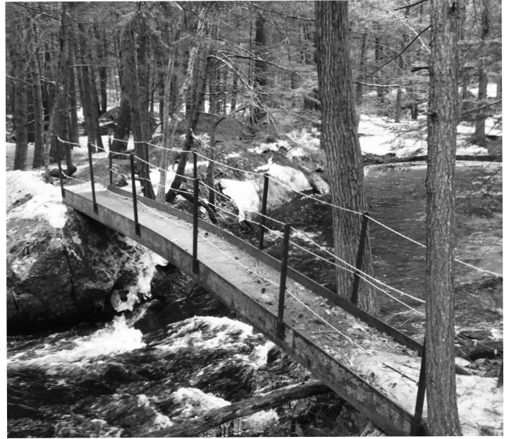
The Webb/Crowell Forest I-beam bridge in Sutton.
